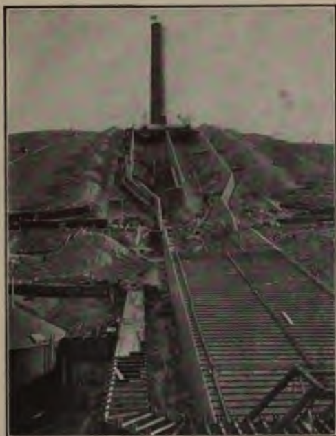
THE SMELTER FLUE AT ANACONDA A VIEW DURING CONSTRUCTION GIVING AN IDEA OF ITS 120-FT. WIDTH AND 20-FT. DEPTH
