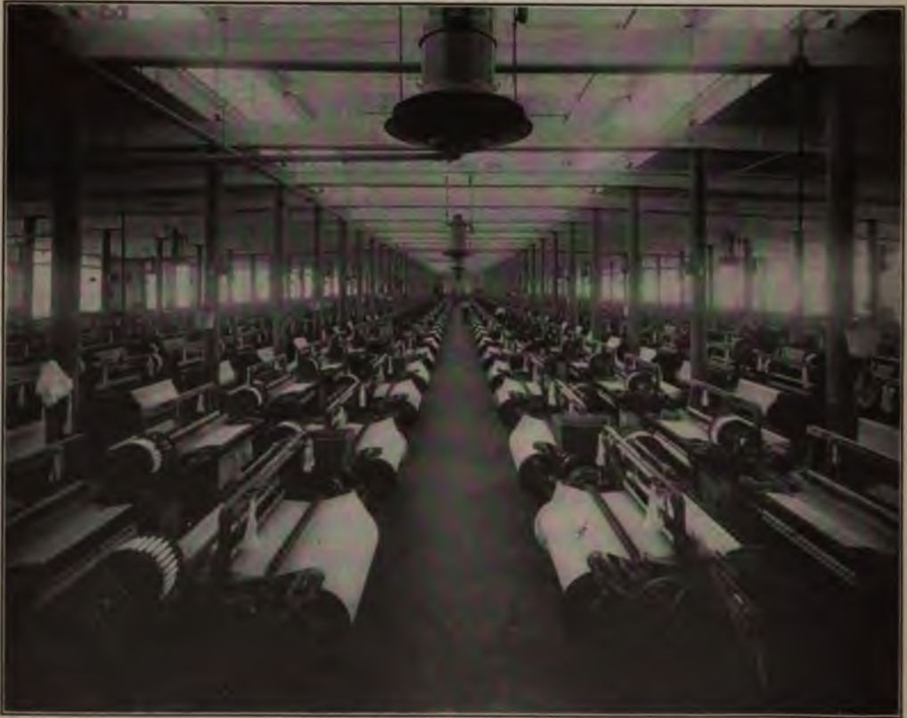
THE WEAVE ROOM OF THE REPUBLIC MILLS
