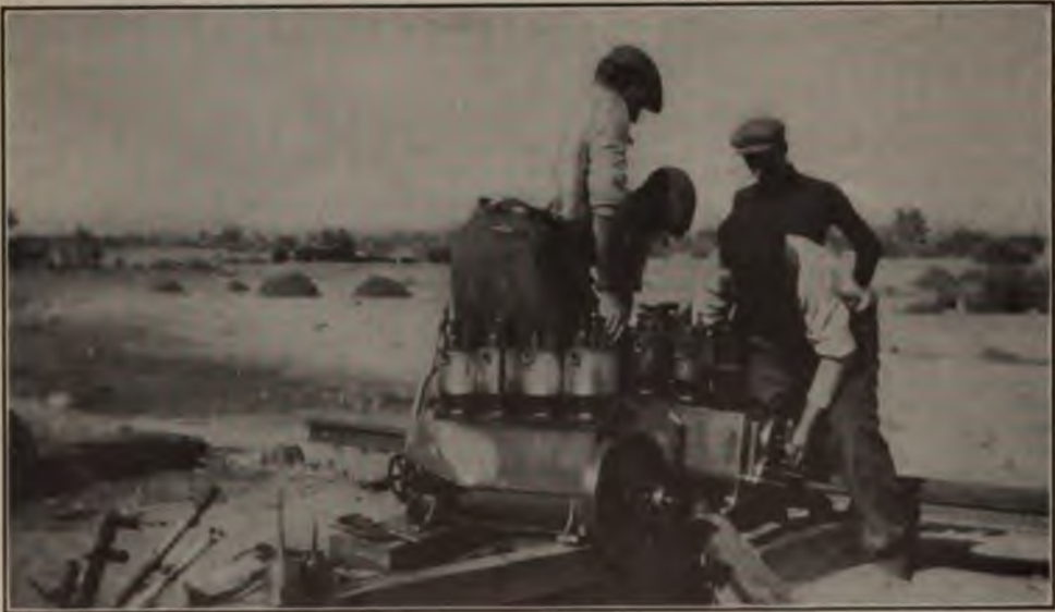
REBUILDING THE ENGINE IN THE DESERT
