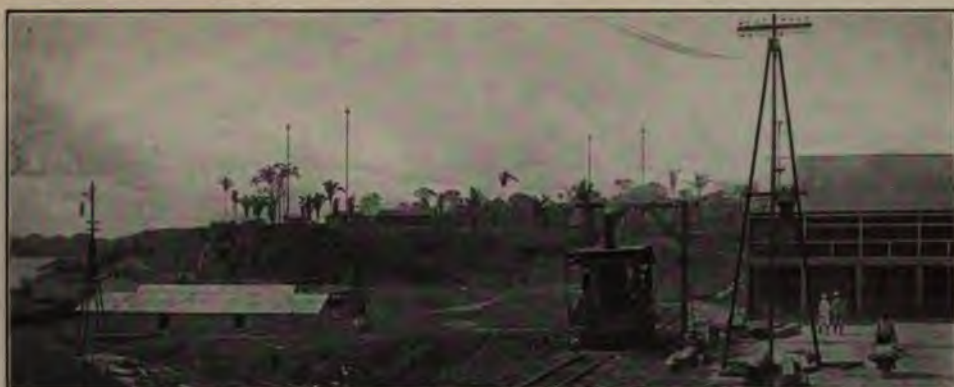
"WIRELESS," IN THE BRAZILIAN JUNGLE AT PORTO VELHO CAPABLE OF TALKING 500 MILES TO MANAOS. ALSO PART OF THE RAILROAD BEING COMPLETED AROUND THE RIBERAO RAPIDS BY AMERICAN CONTRACTORS
