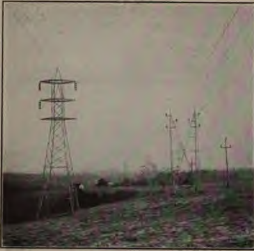
TRANSMISSION LINES OF THE SOUTHERN POWER COMPANY, THE FIRST SYSTEM TO CARRY 100,000 VOLTS LONG DISTANCES
