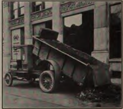
A CONTRACTOR'S TRUCK PARTICULARLY ADAPTED TO BUILDING THE GOOD ROADS WHICH THE COMING OF THE AUTO- MOBILES AND MOTOR TRUCKS DEMAND
