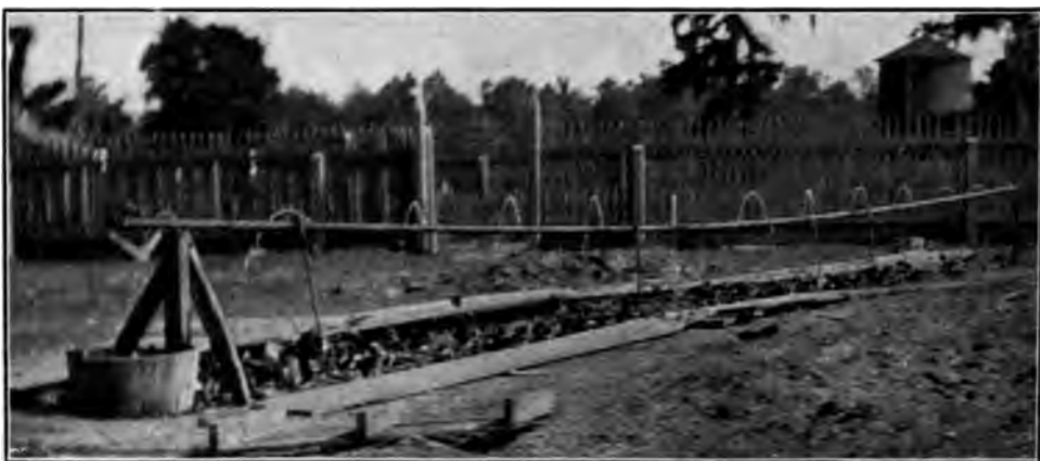
A HOME-MADE SCHOOL FOUNTAIN A CRUDE BUT EFFECTIVE WAY OF ABOLISHING PUBLIC DRINKING CUPS
