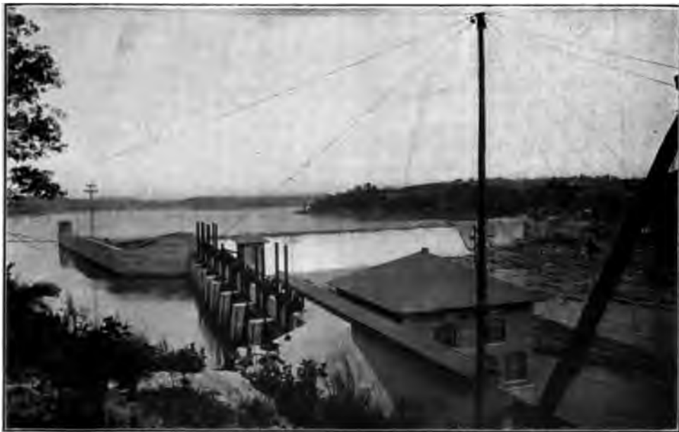
THE ROCKY CREEK, S. C., STATION OF THE SOUTHERN POWER COMPANY WHICH SUPPLIES POWER TO 152 COTTON MILLS, LIGHTS FORTY-FIVE OR FIFTY TOWNS, AND HAS AN EXTENSIVE INTERURBAN TROLLEY SYSTEM UNDER CONSTRUCTION
