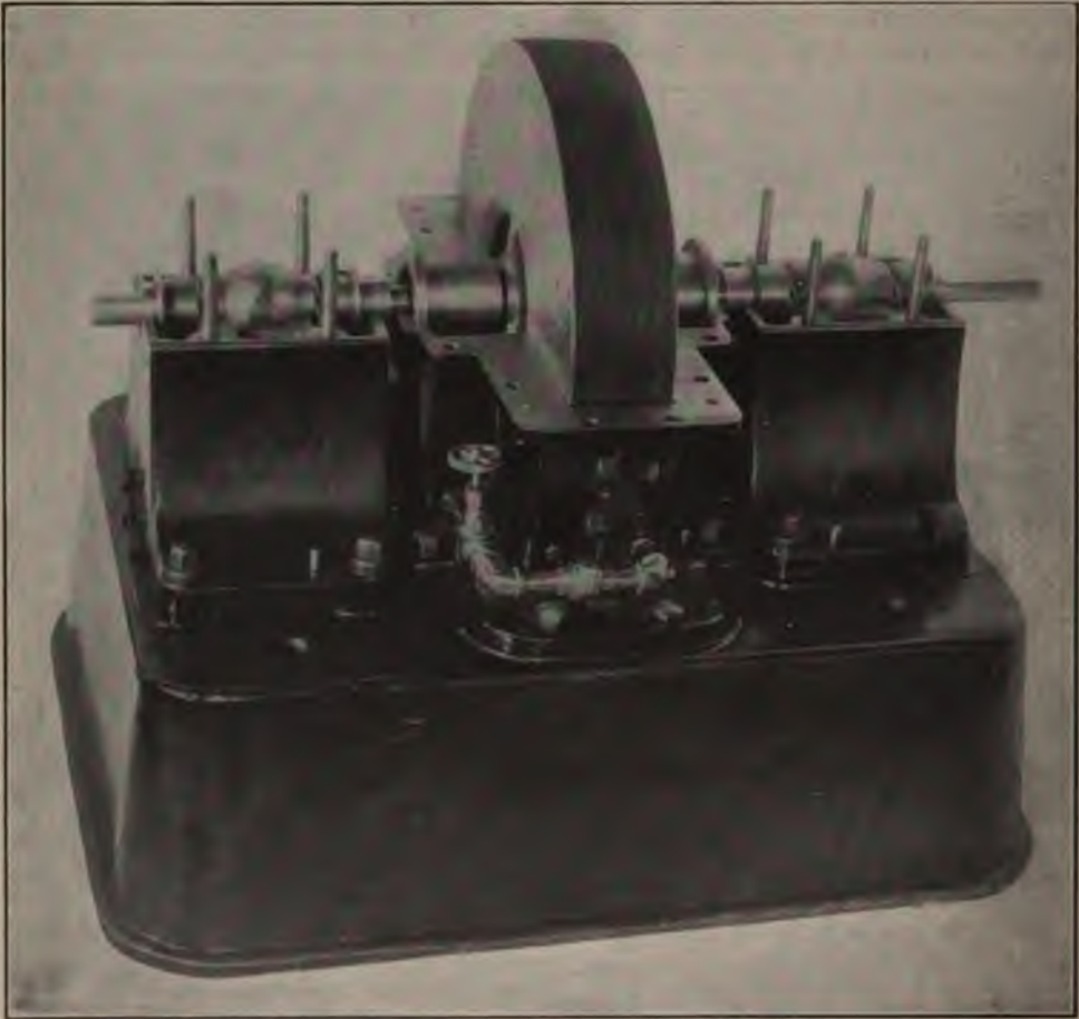
A TESLA TURBINE WITH THE TOP OFF
