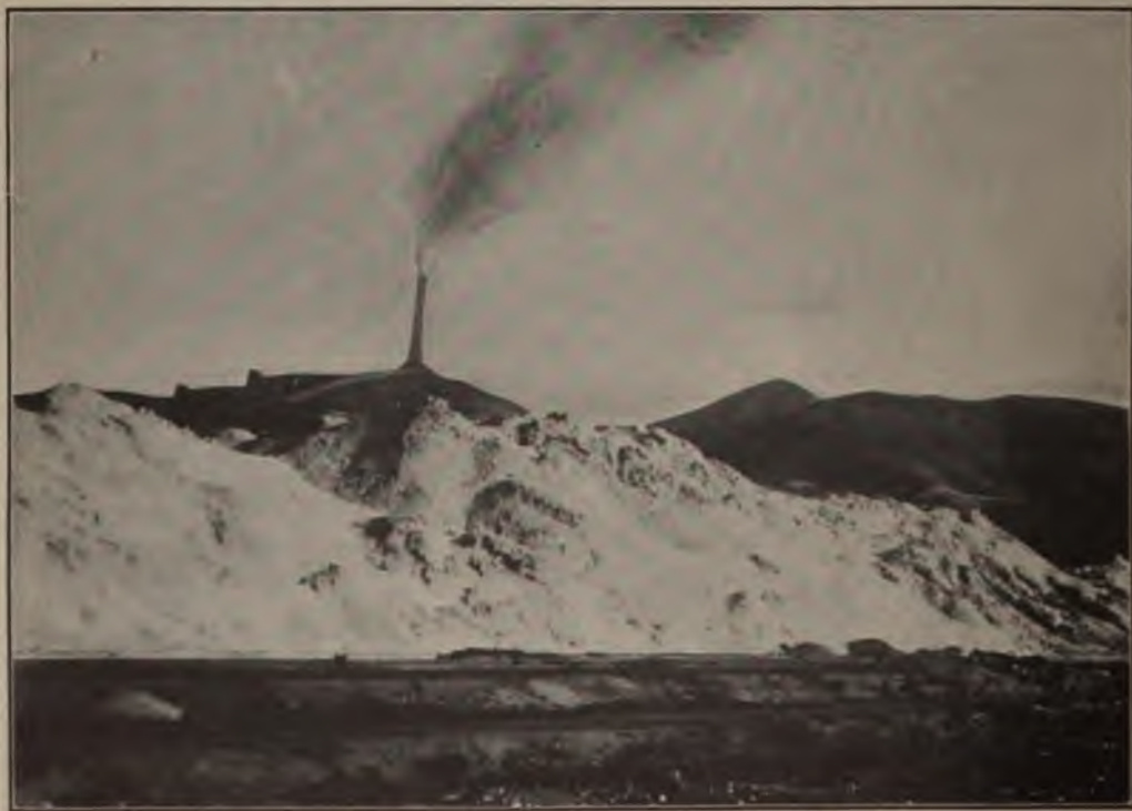
THE GREAT ANACONDA STACK SPREADING FUMES OVER THE COUNTRYSIDE THROUGH THE FLUE LEADING UP TO THIS STACK EVERY DAY PASS GASES CONTAINING NEARLY 30 TONS OF ARSENIC, 2 TONS OF LEAD, 3 TONS OF ZINC, A TON AND A HALF OF BISMUTH, AND ENOUGH SULPHUR TO MAKE 50 TANK-CAR LOADS OF SULPHURIC ACID
