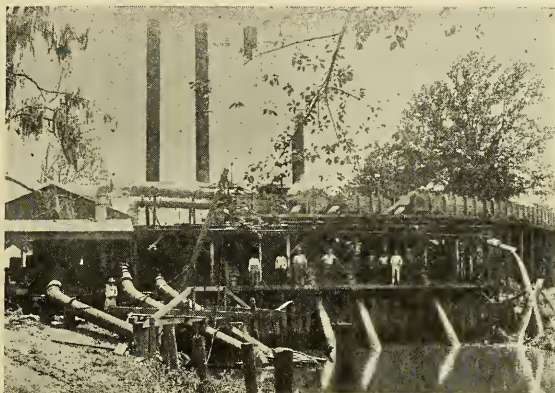
IRRIGATION PUMPING PLANT IN WEST LOUISIANA. —Courtesy of S. Locke Breaux.
