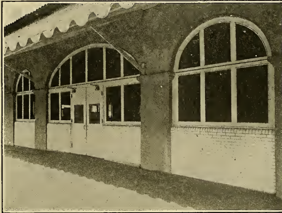
FRENCH MARKET AFTER RENOVATION.
