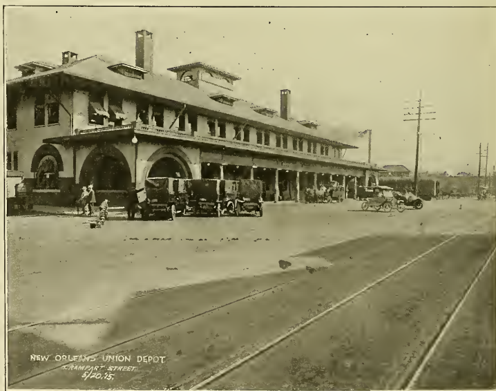
CREOSOTED WOOD BLOCK PAVEMENT.
