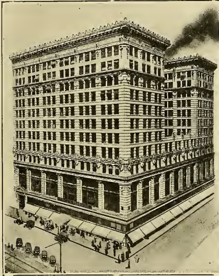
MAISON BLANCHE BUILDING.
