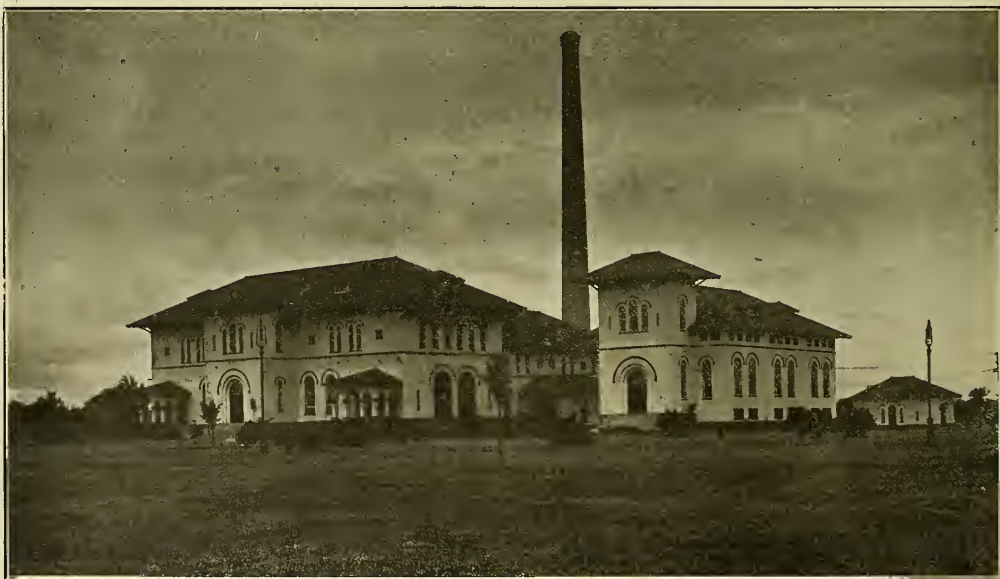
MAIN WATERWORKS PUMPING STATION AND DRAINAGE POWER HOUSE NO. 2.
