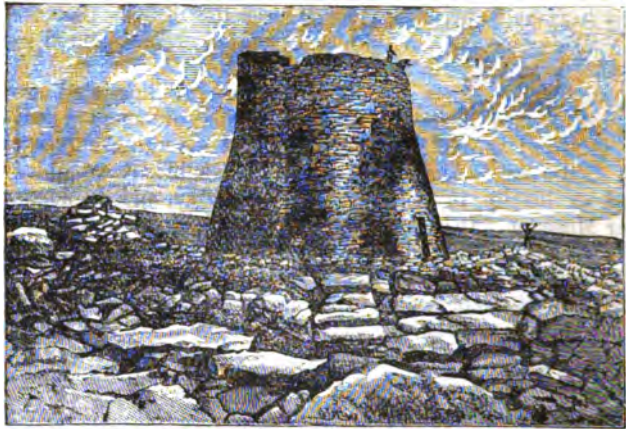
Exterior View of the Broch of Mousa, Shetland.
