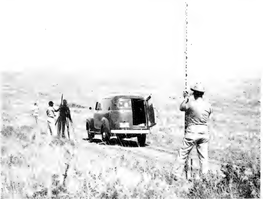
2. A level line party working near Fort Peck, Mont.
