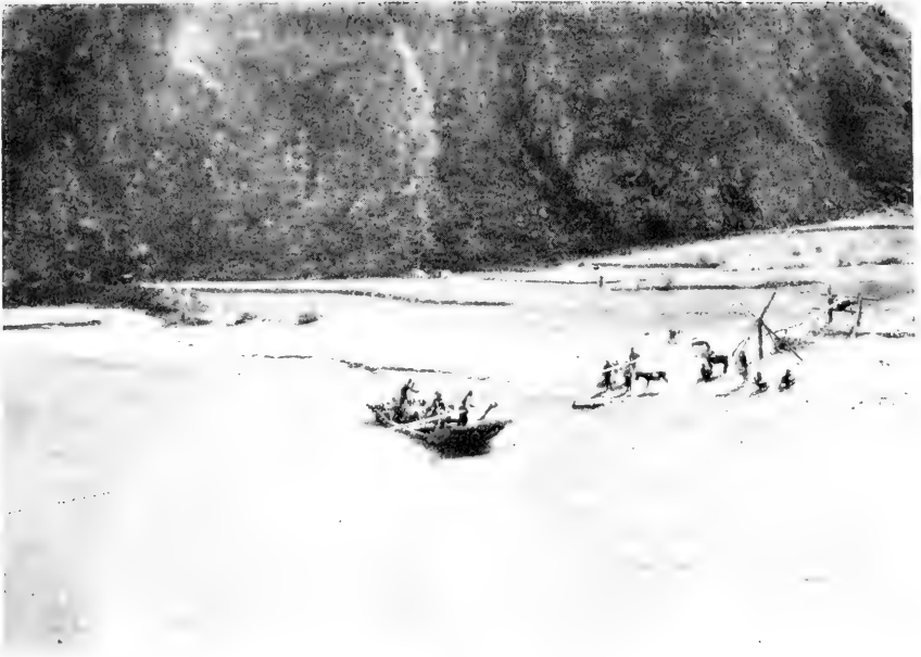
1. Where traffic is light, a costly bridge would be no great improvement over this simple bamboo cable. With the aid of a sturdy hardwood clip, it uses the force of the current to propel the heavily laden ferryboat to and fro across the Siku River on the border of Tibet. (Photograph by F. N. Meyer, from the U. S. Department of Agriculture.)
