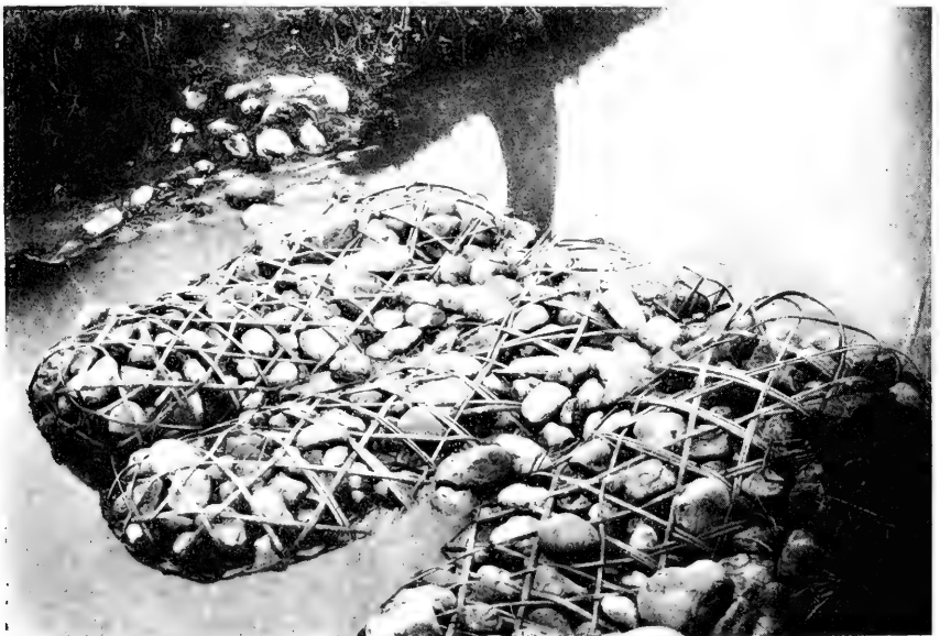
2. Although the bamboo withes from which they are made appear frail and inconsequential, these baskets effectively stabilize a footbridge of field stones near Kao-dien, Hupeh Province, China. (Photograph by F. N. Meyer, from the U. S. Department of Agriculture.)
