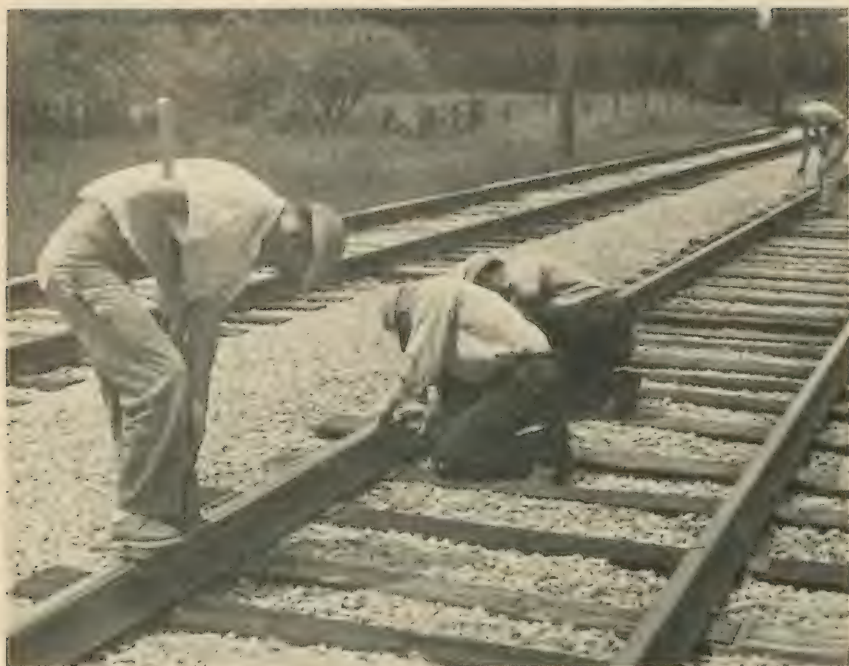
1. Baseline measurement for the triangulation network.
