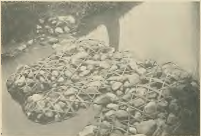
2. Although the bamboo withes from which they are made appear frail and inconsequential, these baskets effectively stabilize a footbridge of field stones near Kao-dien, Hupeh Province, China. (Photograph by F. N. Meyer, from the U. S. Department of Agriculture.)
