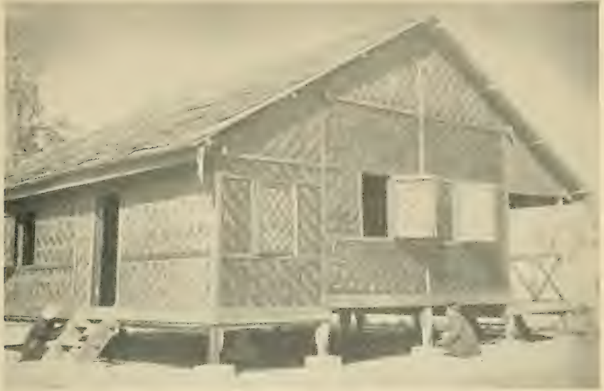
1. Hardwood-framed house with walls of bamboo matting and roof of bamboo shingles ( Bambusa polymorpha ). A modern adaptation developed in Burma.
