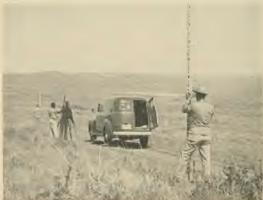
2. A level line party working near Fort Peck, Mont.
