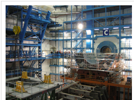
ATLAS experiment detector under construction in October 2004 in its experimental pit; the current status of construction can be seen on the CERN website. [4] Note the people in the background, for comparison.
